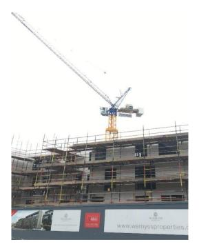
The four upper storeys are constructed in steel frame construction, the exterior cladding is a combination of ashlar stone rain screen and insulated render system with large areas of glass.
