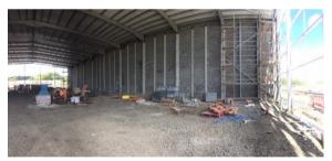
Work was undertaken with the existing warehouse stock left in place. A temporary protection was achieved by hanging a fire blanket from the existing roof of Warehouse 3&4 and covering the floor with a sand carpet to prevent sparks should a block or tools be accidentally dropped.
